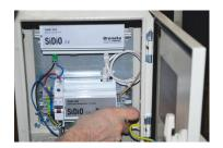
We are placing to the district heating substation a module for remote control "SiDiO'. After that, with the use of a special software we are establishing remote access to the station in order to optimize its workflow.
